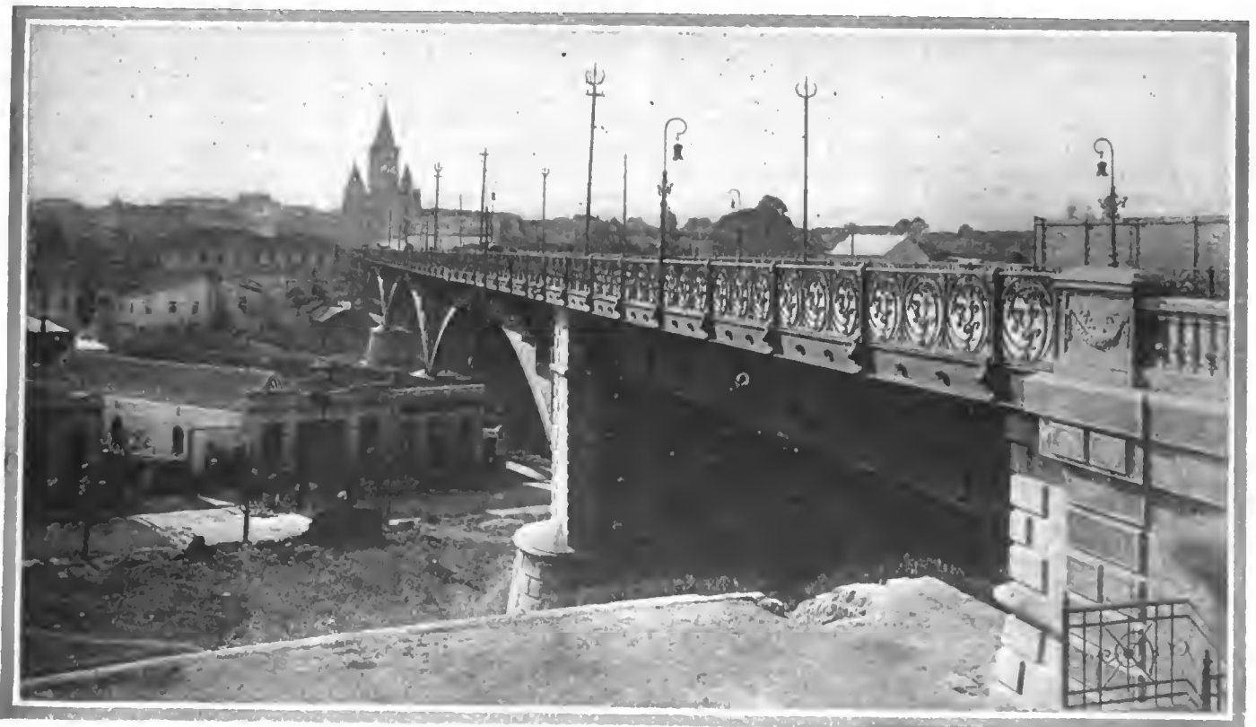
This large viaduct near the heart of the city of Sao Paulo is an example of the enterprising spirit of the city and is indicative of the general go-ahead spirit of the state of Sao Paulo. This viaduct carries double street car lines and is amply wide for all kinds of traffic in both directions. When you find a city adding street improvements of this nature you are certain it will be a profitable motor truck market
